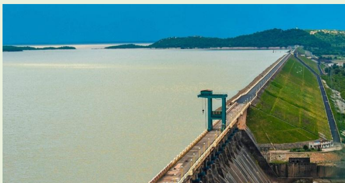
Hirakud Dam, Sambalpur
